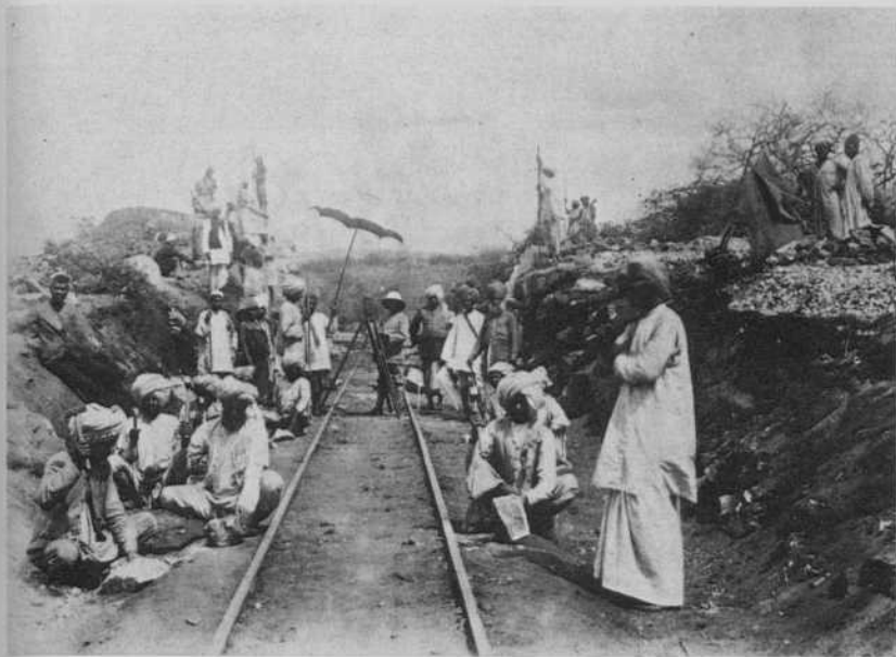
20 Railway builders: Indian coolies laying the track
